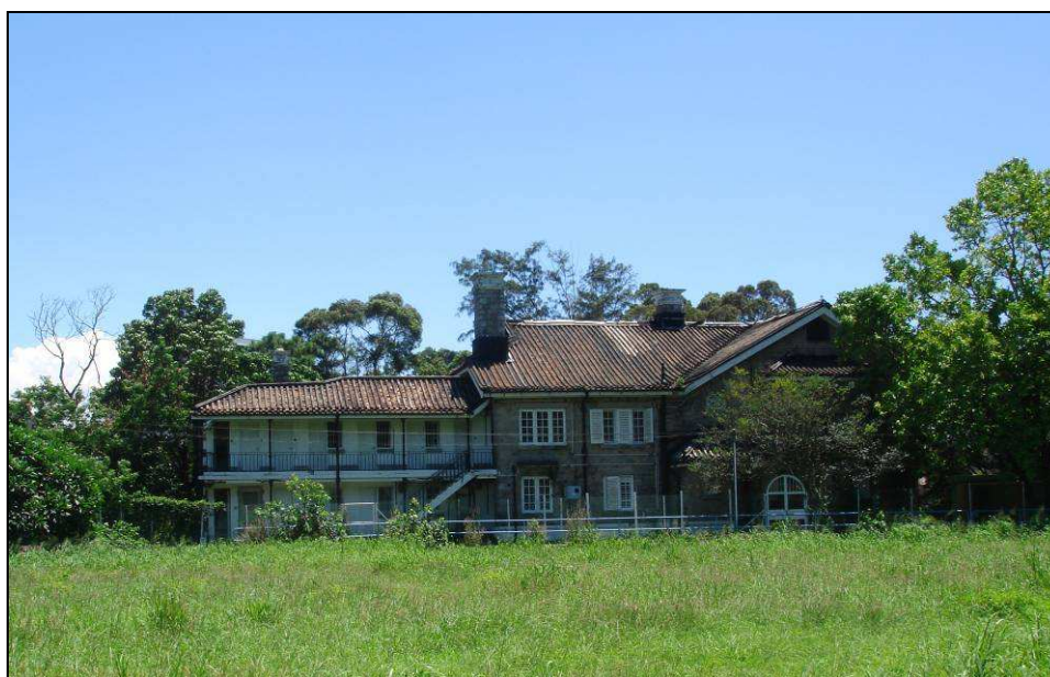
Plate 1 – Elliot Pumping Station and Filters, Senior Staff Quarters (Senior Staff Quarters)
