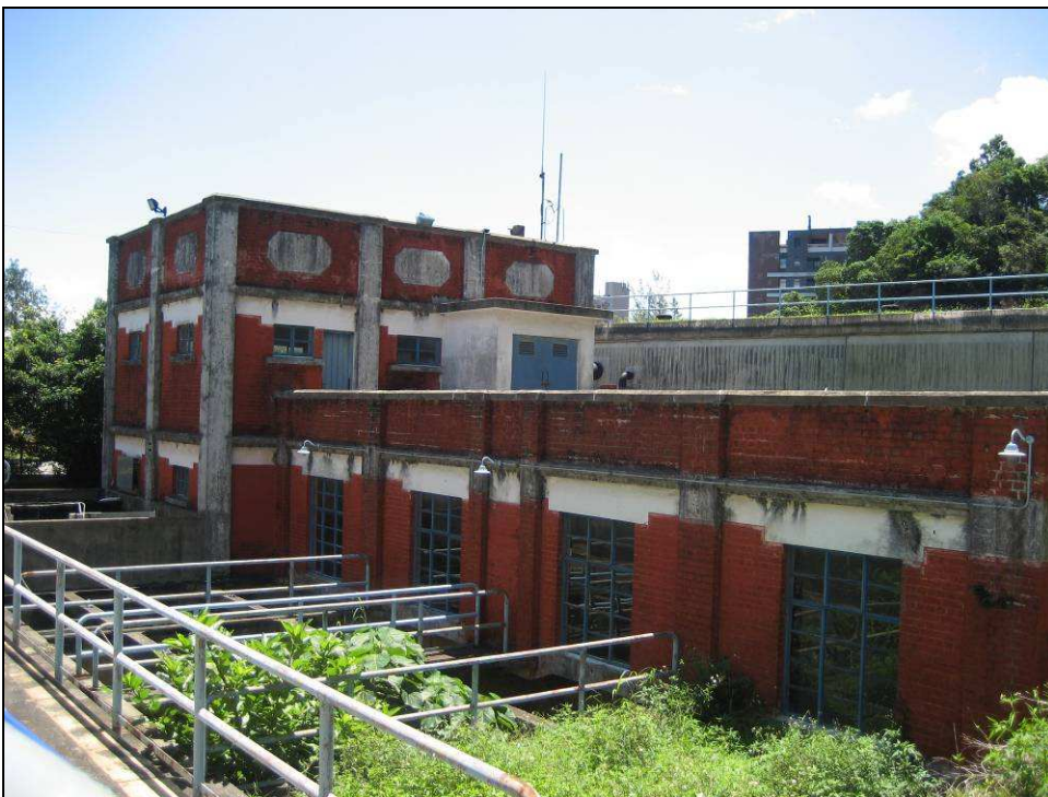
Plate 3 – Elliot Pumping Station and Filters, Treatment Works Building (Treatment Works Building)
